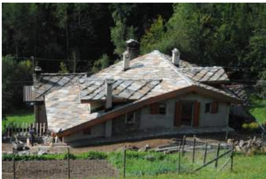
Intervento in Borgata Reynaud
